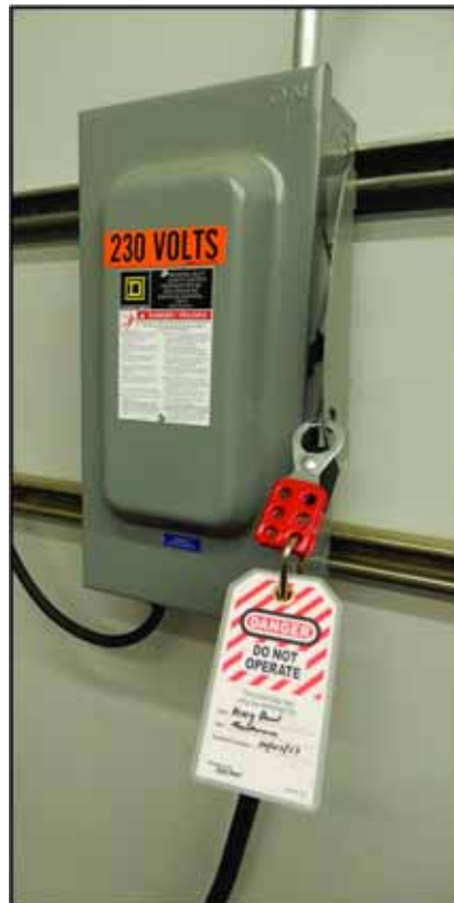
Figure SAFETY-2: Sample of a Lockout/Tagout Mechanism on an Electrical Service Entry Panel
