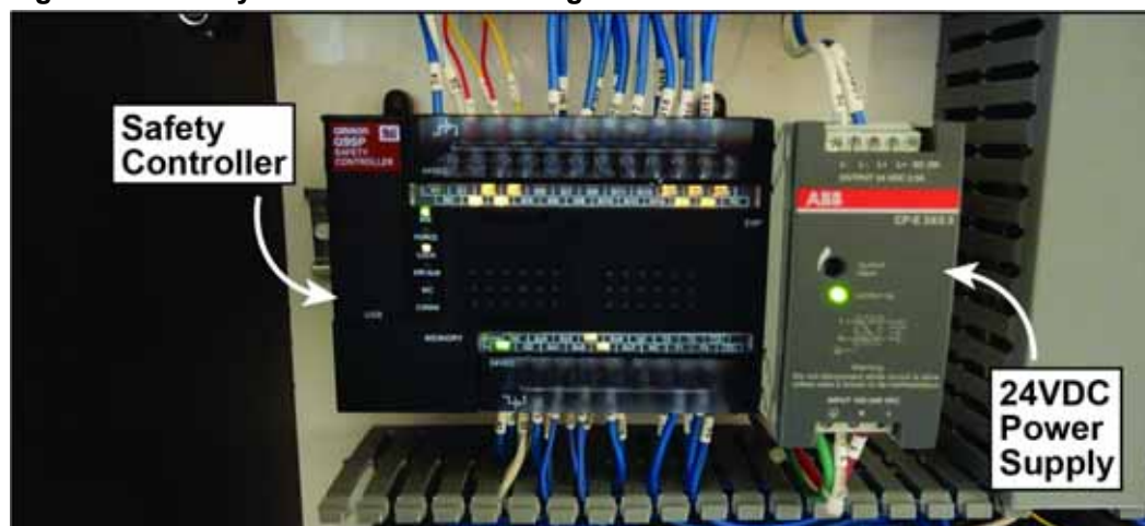
Figure 5-3: Safety Controller Indicator Lights
